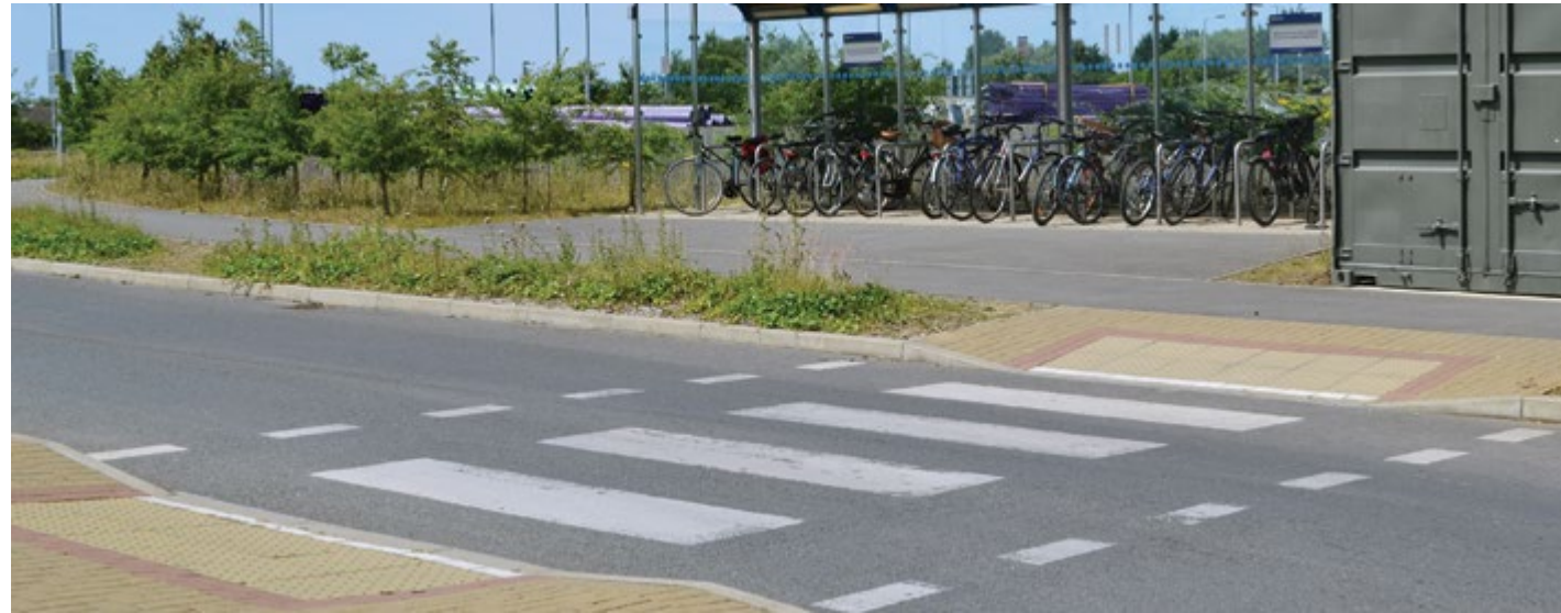
Figure 13 | Curb ramps perpendicular to the curb
