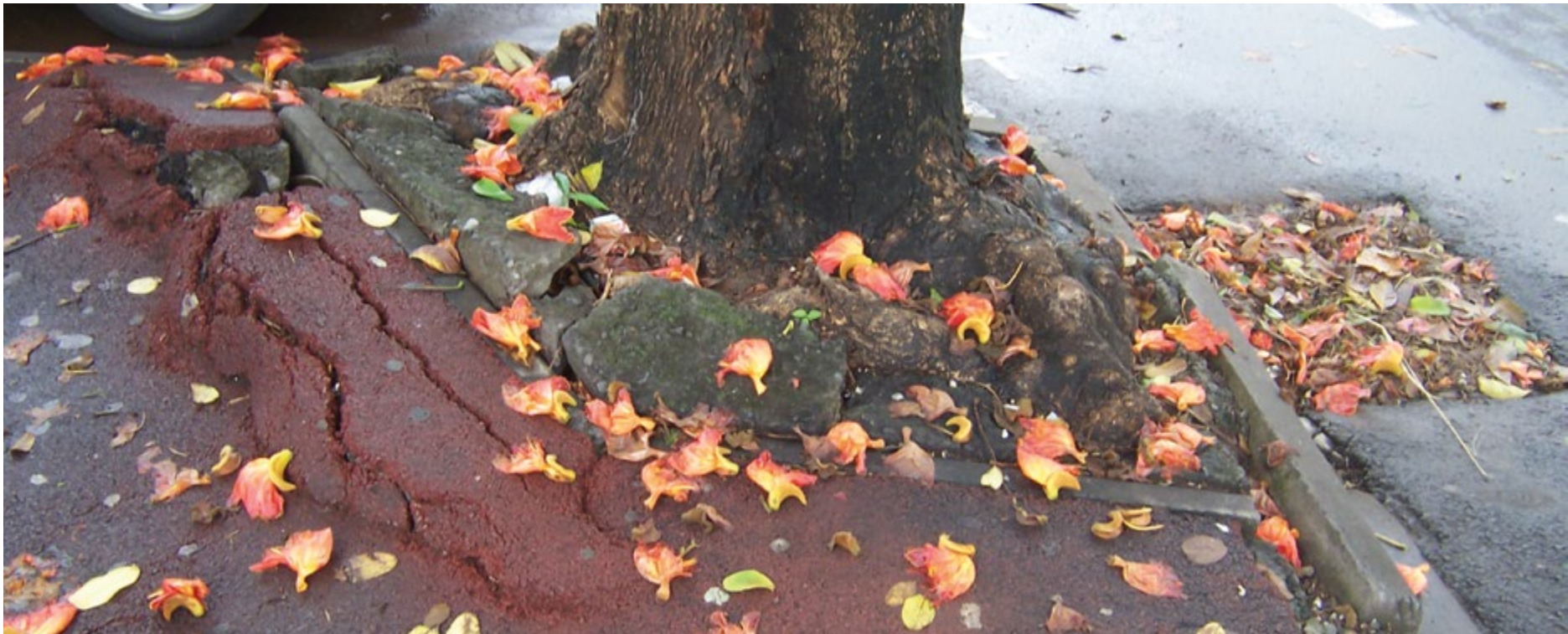
Figure 32 | Sidewalk surface damaged by tree roots
