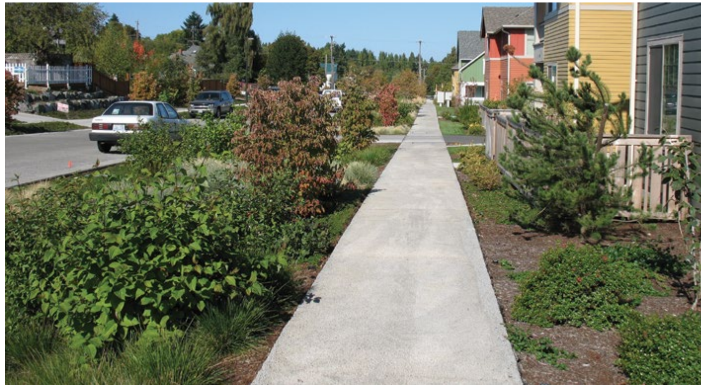
Figure 42 | Sidewalks produced in porous concrete
